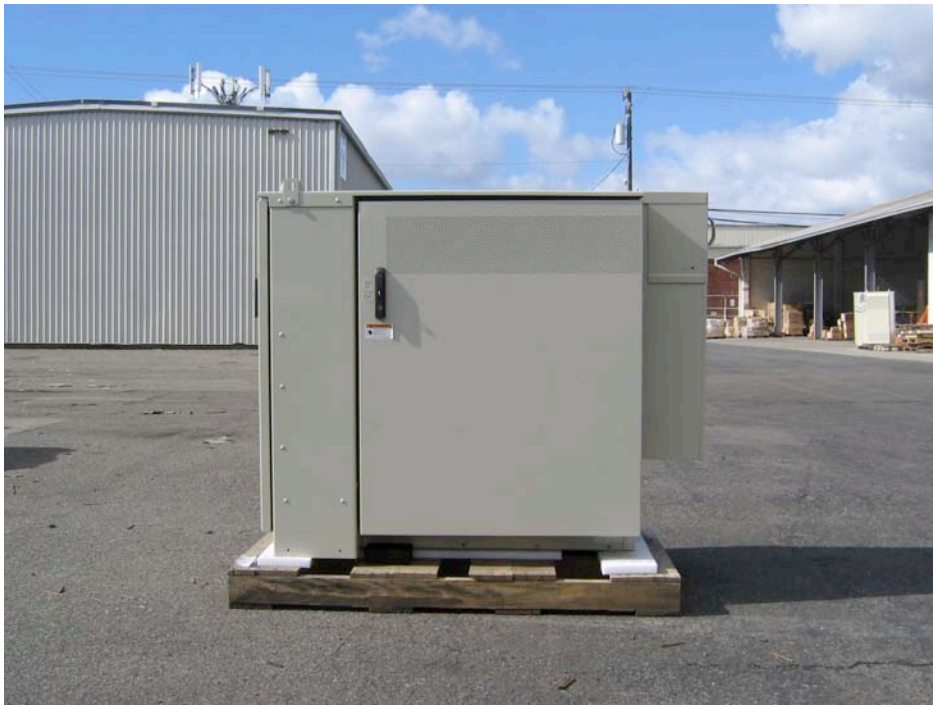
Typical utility box installation for Project Lightspeed
